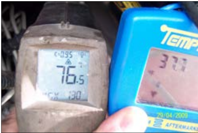
Figure 7: This is a typical reading that can be expected when taking temperature readings on an A/C system with an infrared temperature gun. Both the infrared gun on the left and the contact type temperature reading tool on the right are reading the temperature on the same metal suction line about 1/2-inch apart. Before doing the test, I felt the suction line with my hand, and it felt like a glass of iced tea. The reading on the contact type temperature reading tool indicates a temperature that would be expected of a glass of iced tea. However, the infrared gun indicates a temperature that is almost 40° higher. This was despite numerous efforts to get an accurate reading with it and was the lowest temperature recorded.
